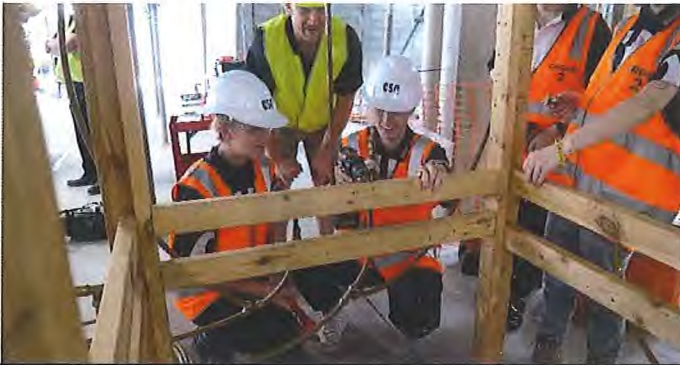
Cannon Hill exemplar project Try a Trade plumbing session TAFE WorldSkills trainer oversees Redlands Vocational College students trying their hands at installing copper pipe
